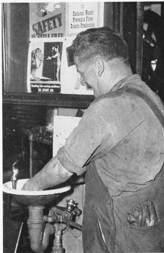
The bubblers are properly serviced whenever necessary by the Pipe Shop. Here Harry Rosevear does a little job. Employees are urged to use the bubblers as drinking fountains — not as sinks — so they'll always be inviting and pleasant.
